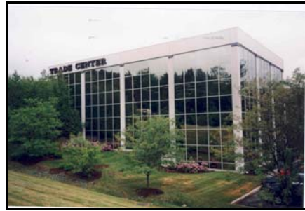
Exterior View from Airport Road
